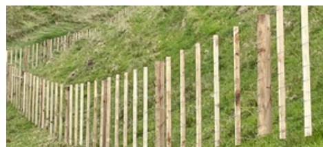
Environmental protection fencing underway
